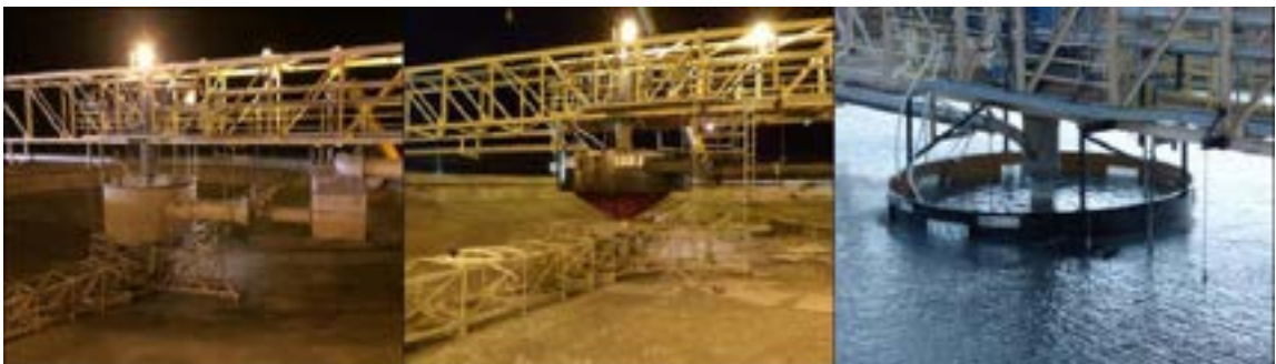
Figure 9: Vector® feed system upgrade to a gold tailings thickener
